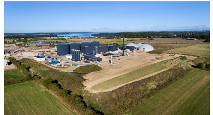
Glansager Biogas – delivers E-methane to the Danish system
