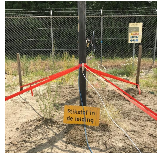
Nitrogen vent DN100 + sample point DNV
