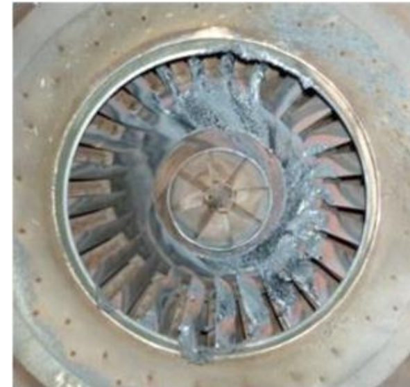
Flashback damage to burners has been linked to high levels of higher hydrocarbons Source: E-ON, David Abbott; EDI Quarterly Volume 4 No 1 April 1012
